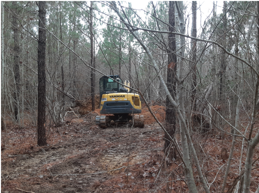
Figure 2: Excavator digging a trench at Argo
